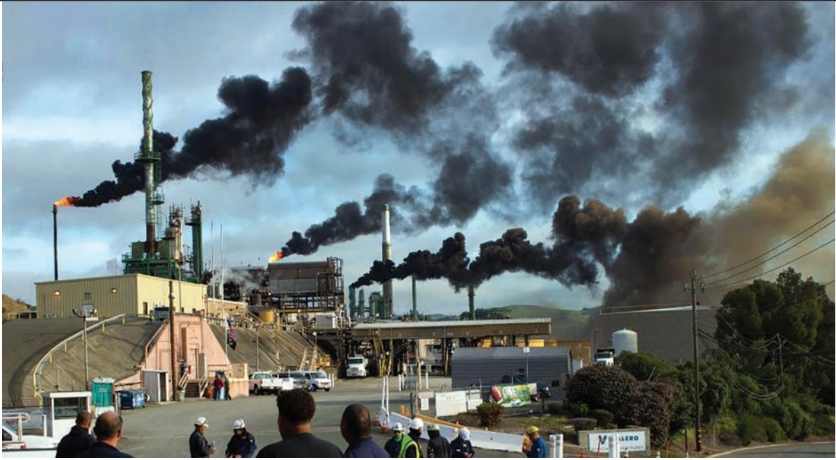
May 5th 2017 Valero flaring incident that forced evacuation of the Benicia Industrial Park.
